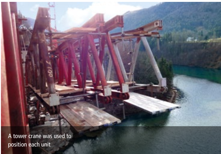
The individual units, each weighing several tonnes, have to be carefully manoeuvred into place to ensure they are installed correctly
