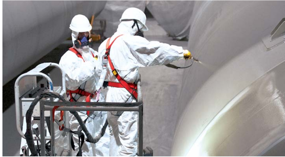
The spray work has to be carried out quickly, as it doesn't take long for the material to set
