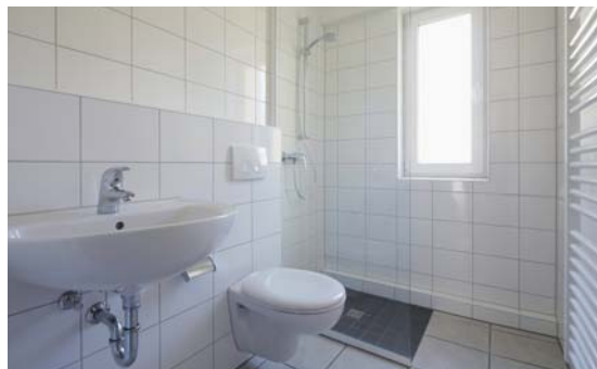
The Thorr estate in Bergheim was fully refurbished – both inside and out – much to the joy of the local residents
