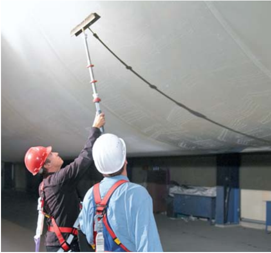
Testing the finished coat for pores using the high-voltage spark test
