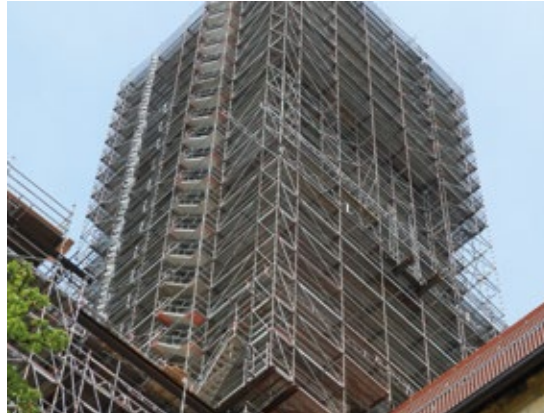
XERVON's scaffolding specialists planned and calculated every section of the scaffolding for the Basilica in Amberg right down to the tiniest of details – an impressive example of their scaffolding expertise
